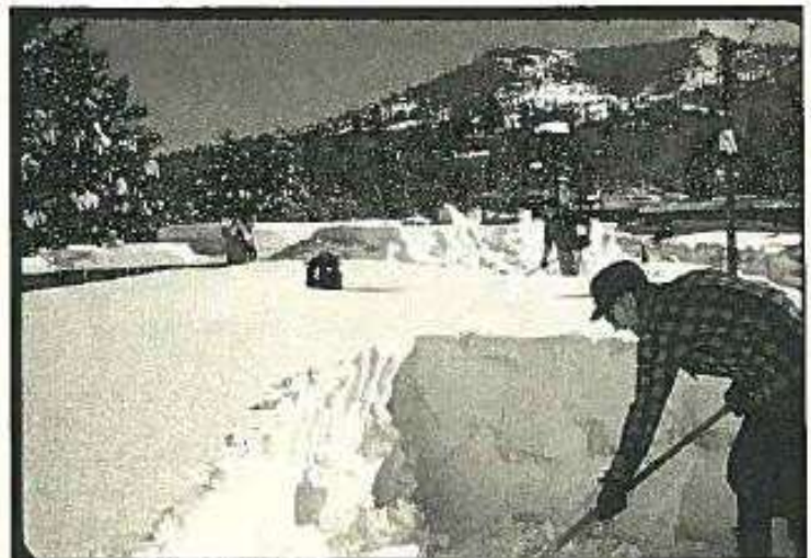
Image 9 – Snow Removal from Rooftops on Gulling Street
