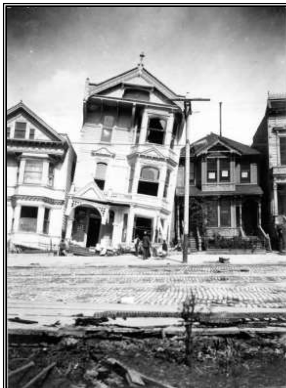
Image 5 – Results of Liquefaction in 1906 ( http://geomaps.wr.usgs.gov/sfgeo/liquefaction/image_pages/tilted_victorian.html )
